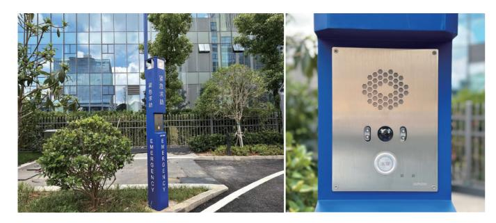
Installed with SPON IP outdoor speakers at factory outdoor public area can be used for playing background music to enhance the cultural atmosphere on a daily basis. Additionally, when integrated with cameras, it can enable alarm linkage for security purposes.
